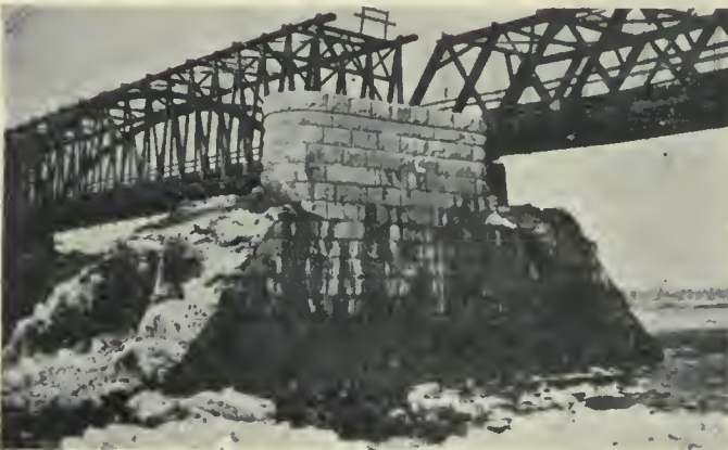
Fig. 3.—Pier No. 4 completed.
